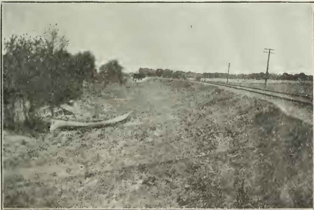
C. East Approach to Bridge. C. & N. W. Ry. Bridge and Approach at Freeport.
